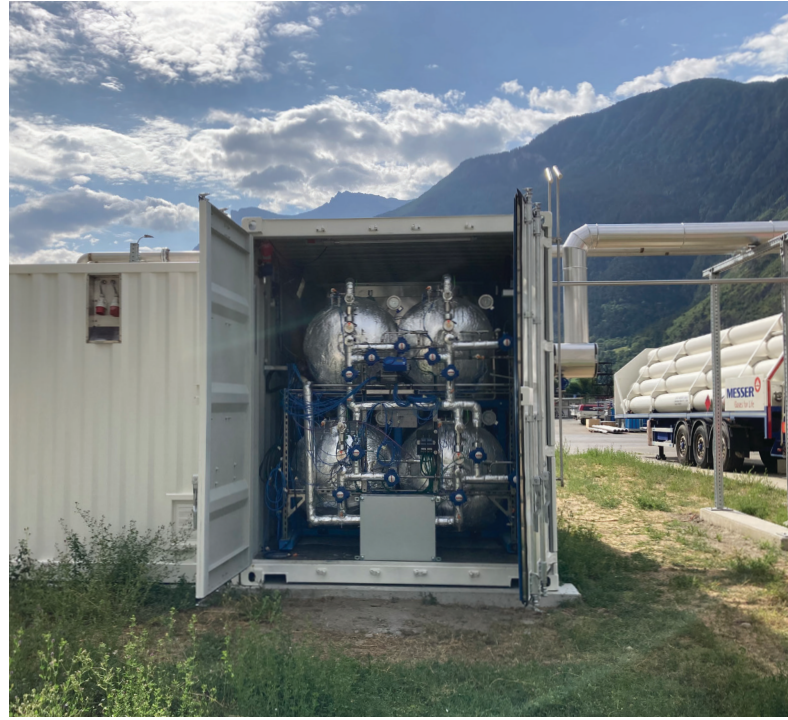
CH-030: Industrial-Scale Metal Hydrides Hydrogen Compressor HyCo
